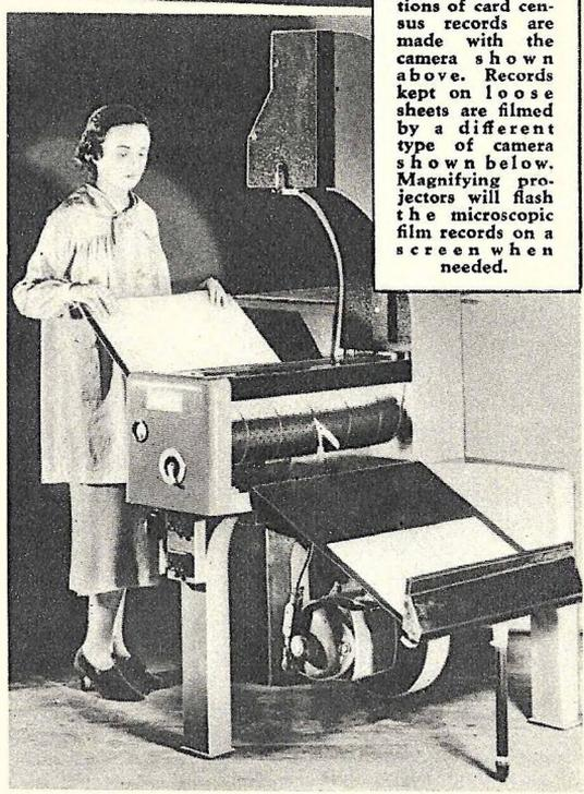
**S**PECIALLY designed giant cameras are being used by the Bureau of the Census to record on motion picture film, in microscopic size, the 126 million names and other data gained in the censuses of 1880 and 1900 which have been kept on cards and in 25-pound volumes occupying a mile of shelves. A 95% saving in storage space will be achieved and the data can be reproduced on a screen, when needed, through use of a magnifying projector.
