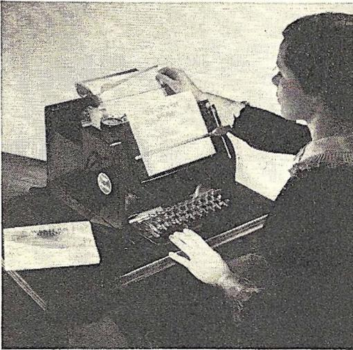
Light weight, noise absorption, and reduced fabricating cost are features of this new molded plastic Western Union Teleprinter housing developed by the General Electric Company.
