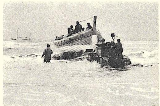
Pushing heavy life boats over sand for launching is eliminated by Netherlands Coast Guard units by using special tractors and trucks to push boats into the surf until they float.
