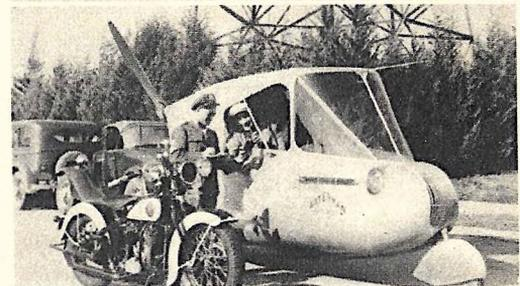
Top—New Arrowbile ready to fly. Below—Wings detached and ready for operation as an automobile. Using a Studebaker engine, the vehicle is capable of a 70-mile-an-hour land speed.
