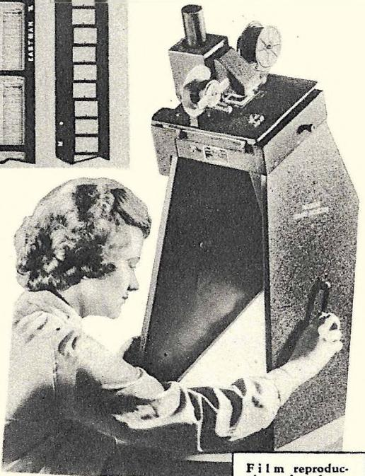
Film reproductions of card census records are made with the camera shown above. Records kept on loose sheets are filmed by a different type of camera shown below. Magnifying projectors will flash the microscopic film records on a screen when needed.
